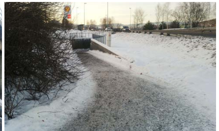
Undergang under E 134
